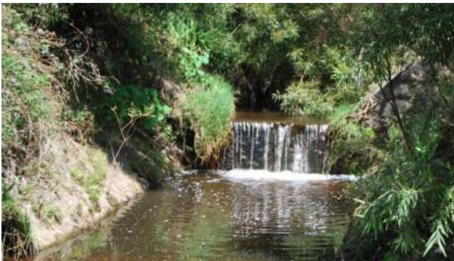
Figure 11: Drop structure on Yakamia Creek in section D2.5
