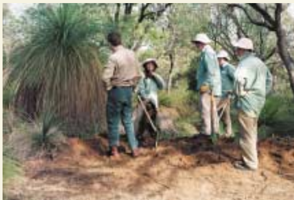
Green Corps team starting to remove the soil dump .
